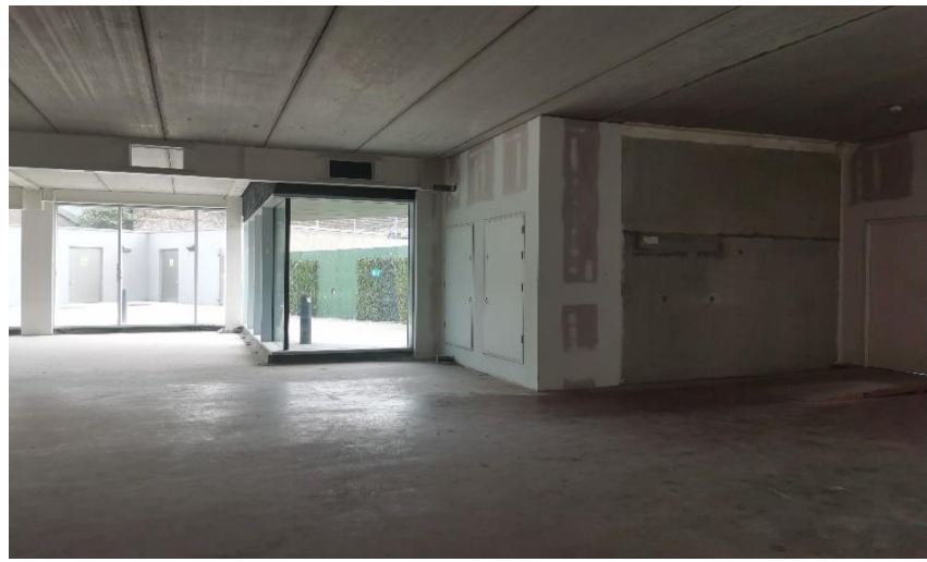
Figure 6.8 Ground floor of Navigation Square building in ‘shell and core’ condition (May 2025)
